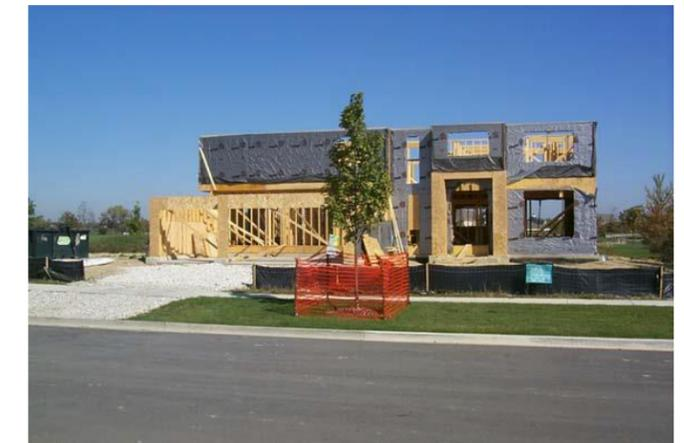
Erosion control is important even for home sites less than an acre. The materials (straw, silt fence, stakes, gravel, plastic tubes, and grass seed) are easy to find and relatively inexpensive. Putting these materials to use is a straightforward process. Only a few controls are needed on most home sites.
